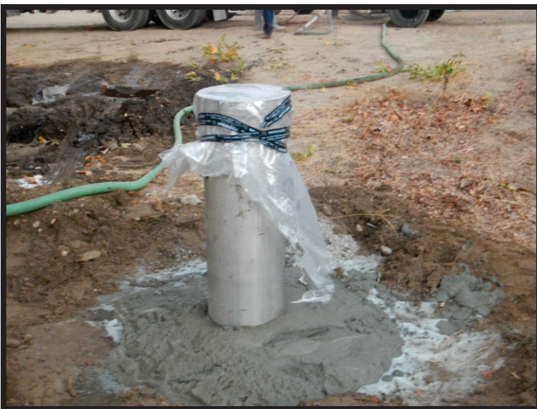
6: The completed well with cement seal showing at the surface.
