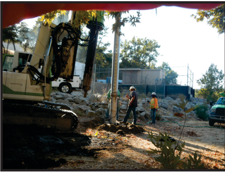
4: Installing the stainless steel screened interval.
