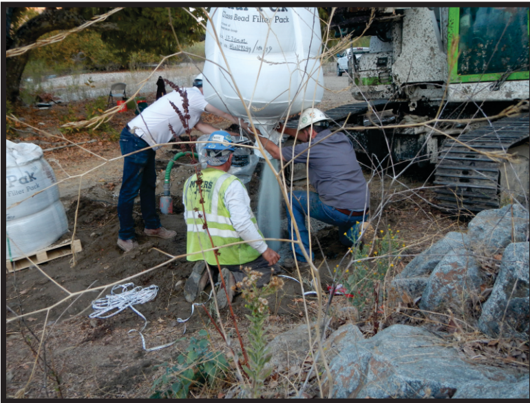
5: Placing the glass bead filter pack.
