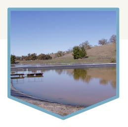
The treatment plant provides secondary treatment through a lagoon/ponding system with a permitted capacity of 0.4 million gallons per day (MGD).
